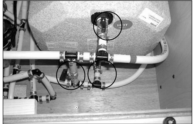
Picture G-P14: Summer mode valve positions.
